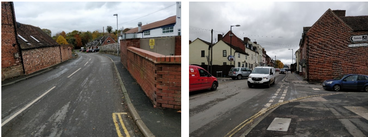
Figure 7: Tenbury Road junction illustrating lack of pedestrian footways
